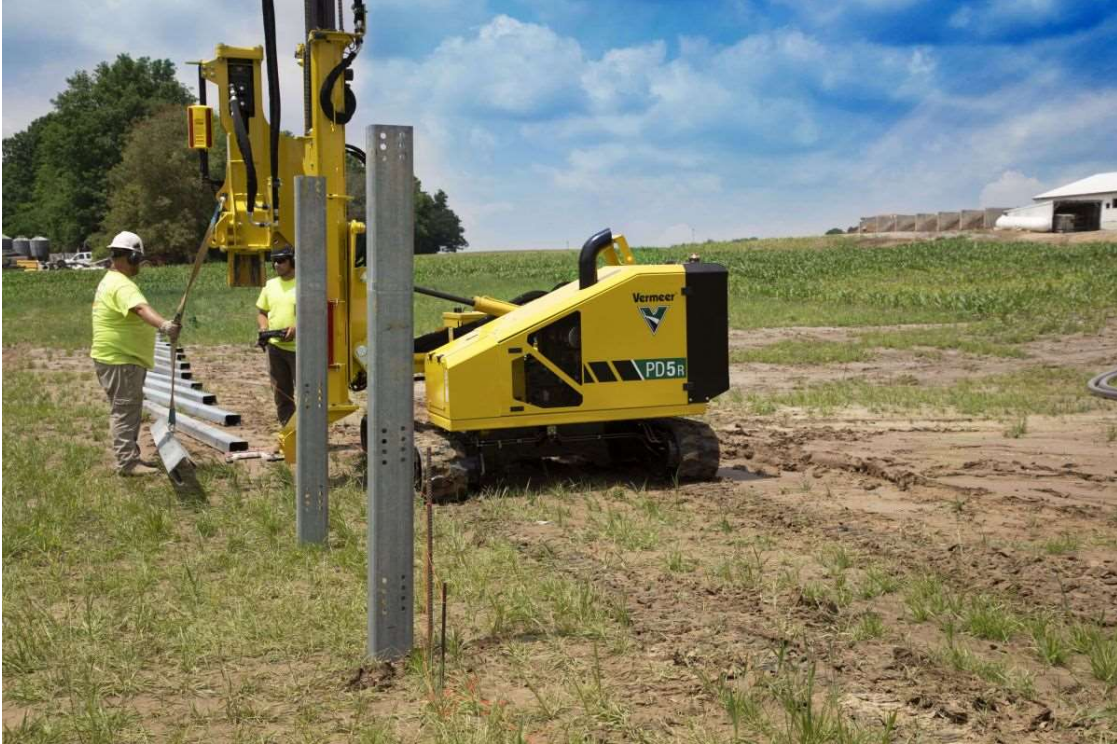
Image 1: Vermeer Pile Driver and construction crew installing solar piles
