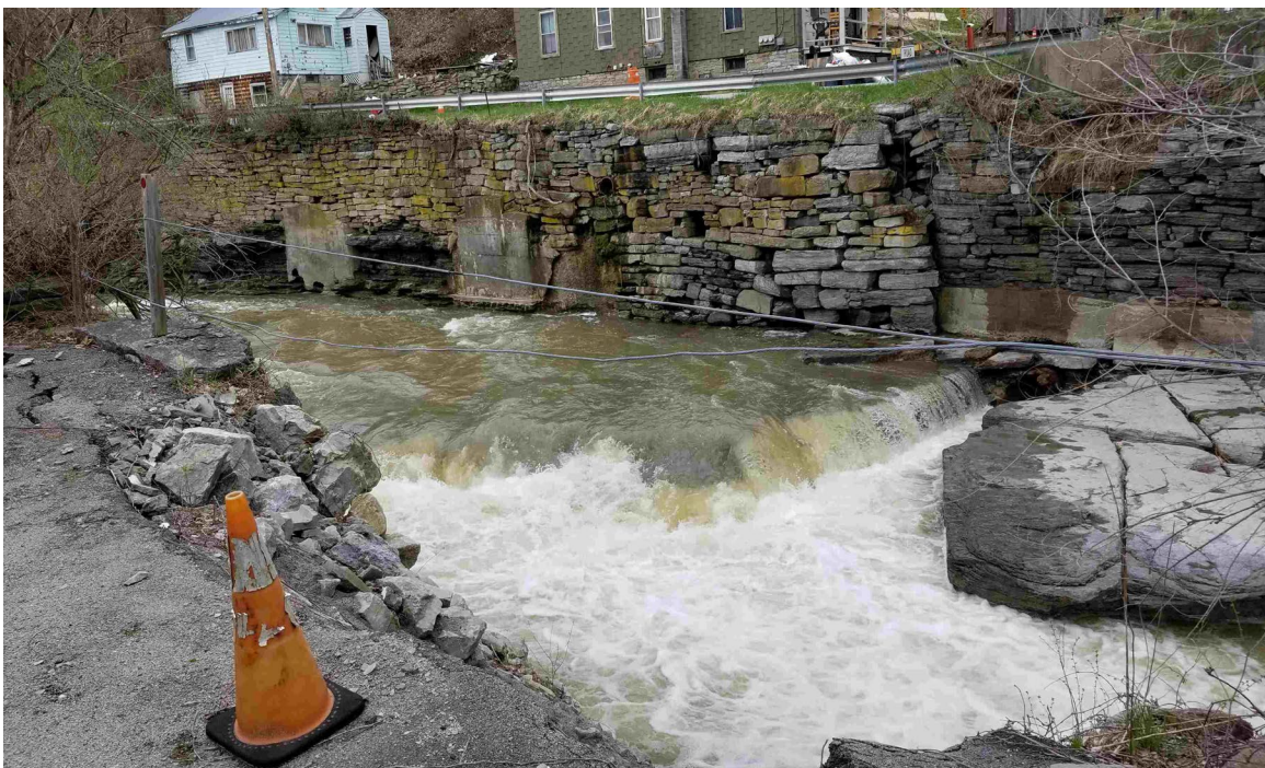
A collapsing section of the retaining wall along the Canajoharie Creek near Mill Street (2019)
