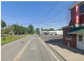
Large setback and curbcuts erode traditional character.
