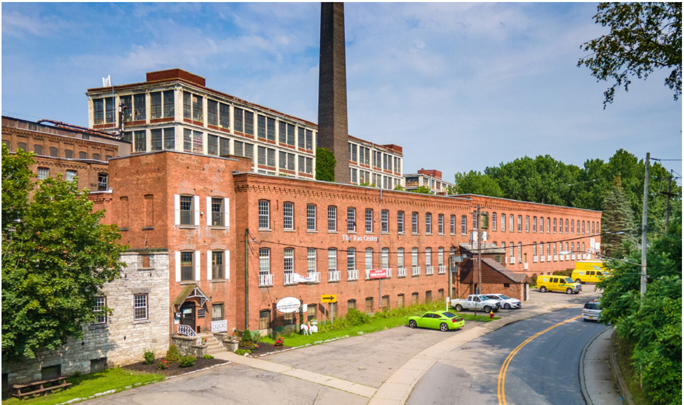
Industrial uses on Church Street.
