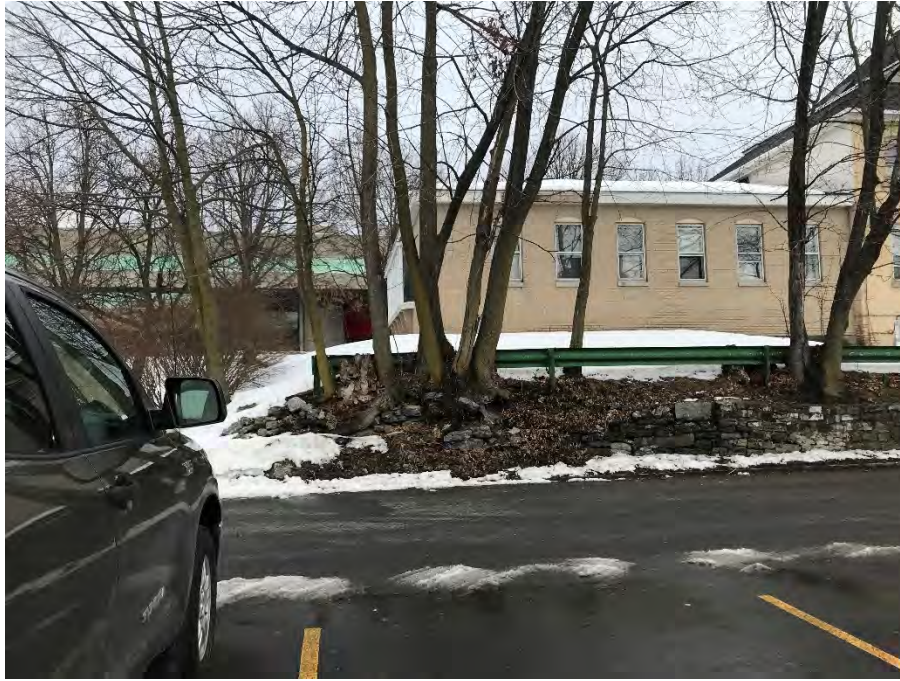
Picture #5: Standing South of Building and Looking N
