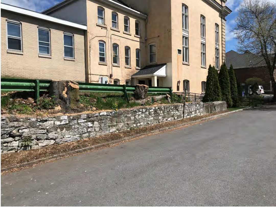
Picture #1: Standing South of Building and Looking NE
