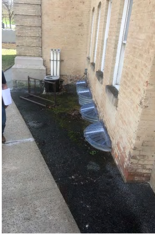
Picture #3: Standing North of Building and Looking E
